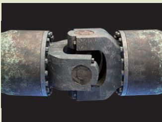
Photo showing condition of U-joint after operation
